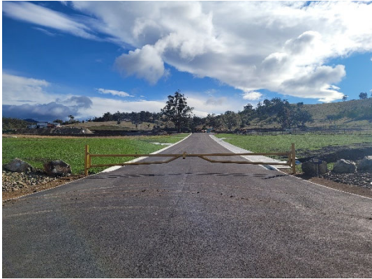
Figure 6 Looking west up the existing road, lots to the right
