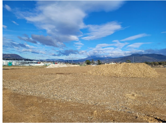
Figure 7 Looking south from the new road opposite lot 3
