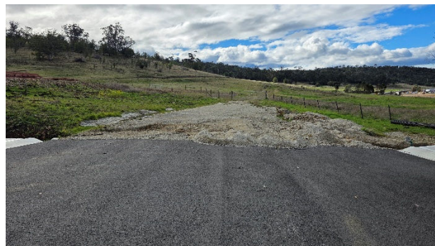
Figure 11 Looking north over lots 2 and 3
