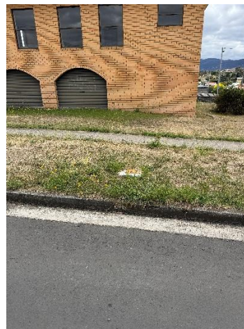
Figure 6.1 – Ex hydrant (west most hydrant on William St)
