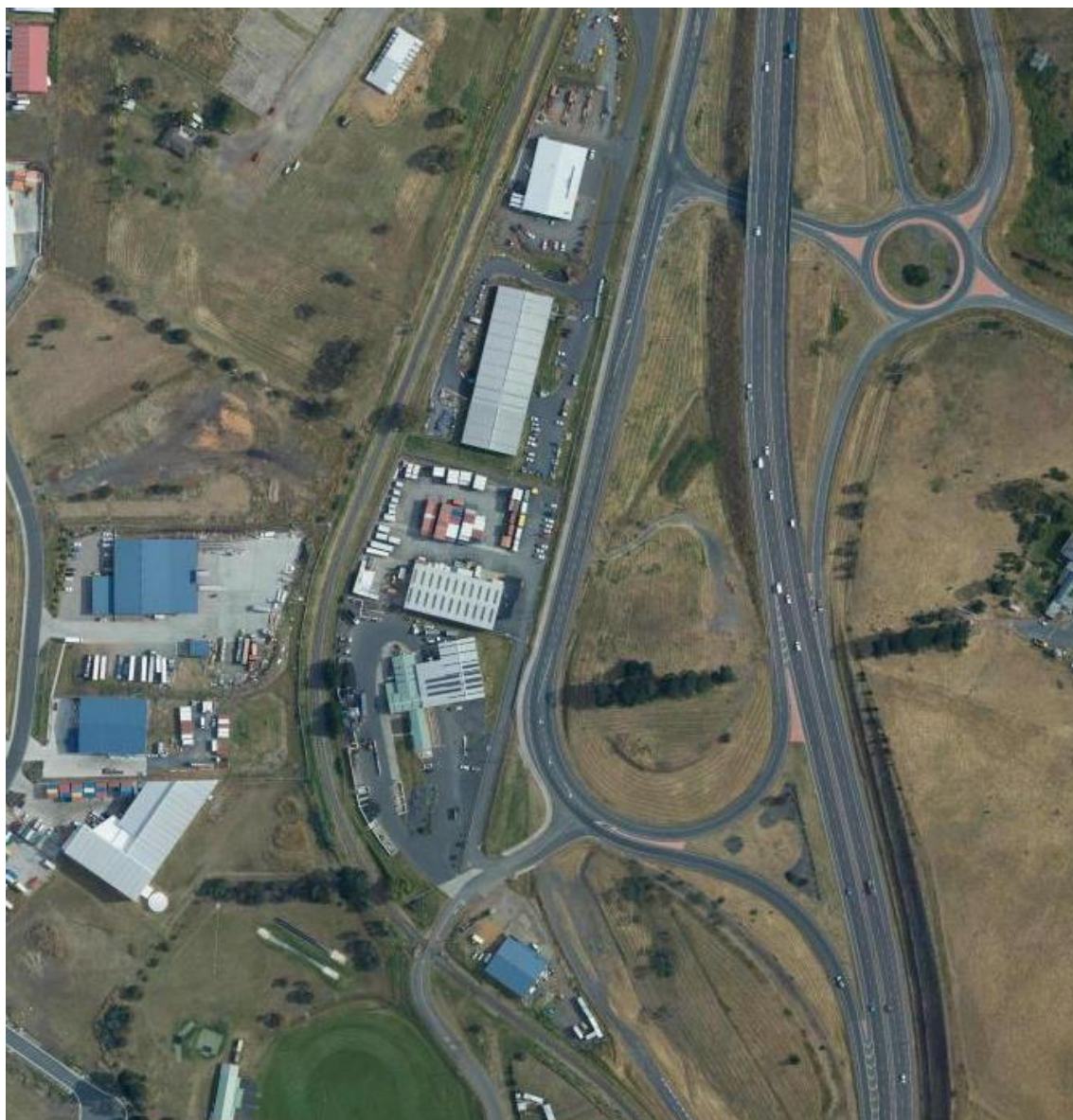
Figure 9 – Midlands Highway / Glenstone Road Interchange – South
