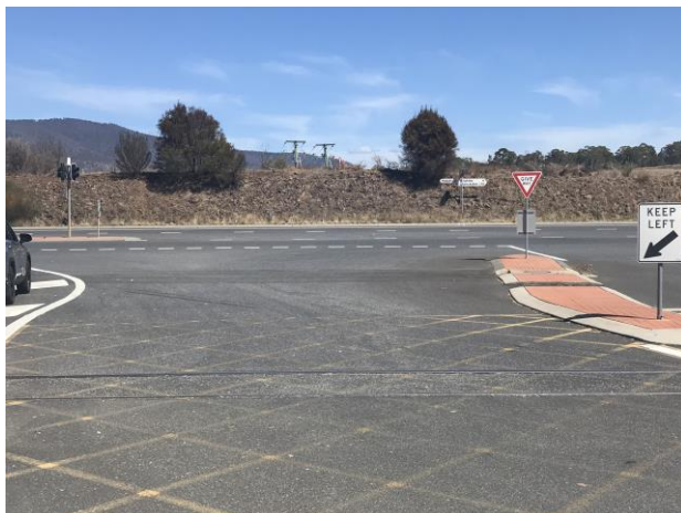
Figure 17 – Brighton Hub Truck Exit approach to Glenstone Road
