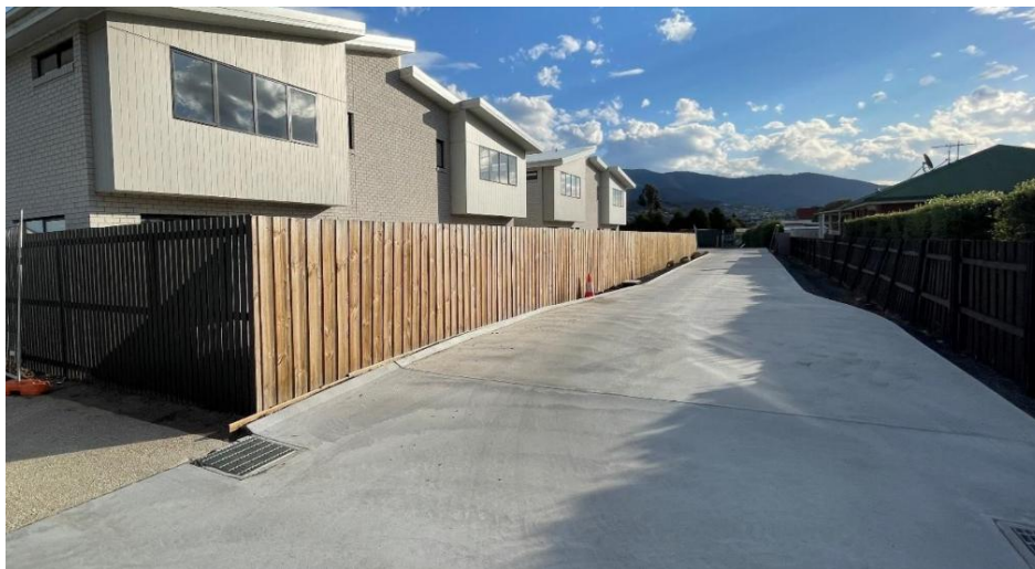
Figure 12: Corner in the internal driveway leading to the second section of access to the site
