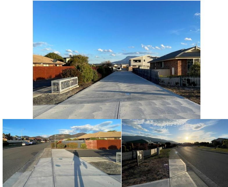
Figure 11: Site entrance and available sight distance
