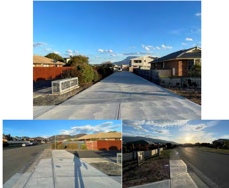
Figure 11: Site entrance and available sight distance
