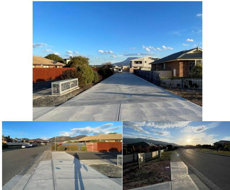
Figure 11: Site entrance and available sight distance
