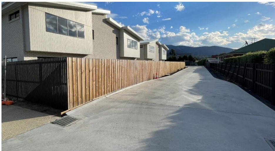
Figure 12: Corner in the internal driveway leading to the second section of access to the site
