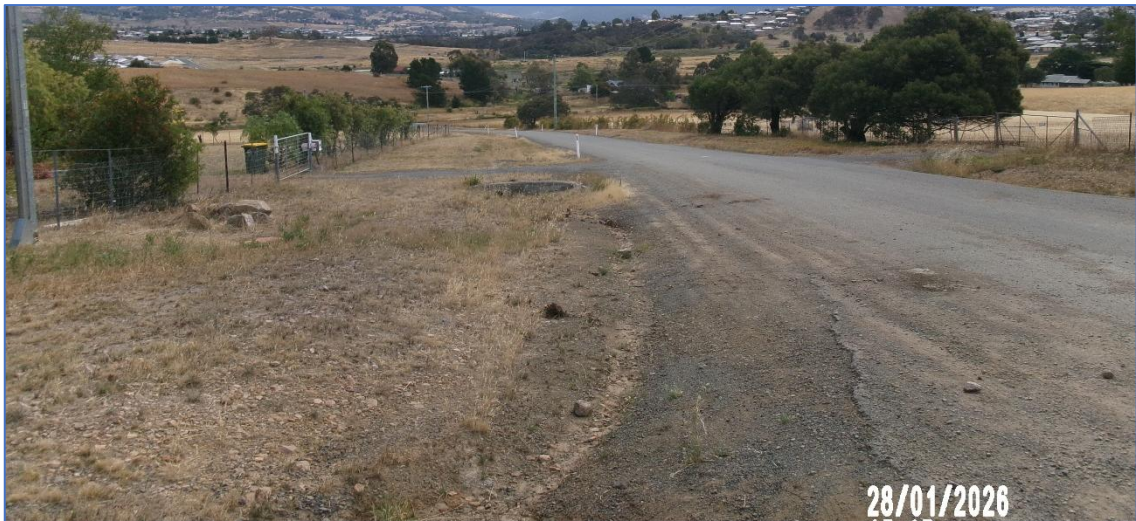
Photograph 7.2A – View for driver leaving the development site to the left
