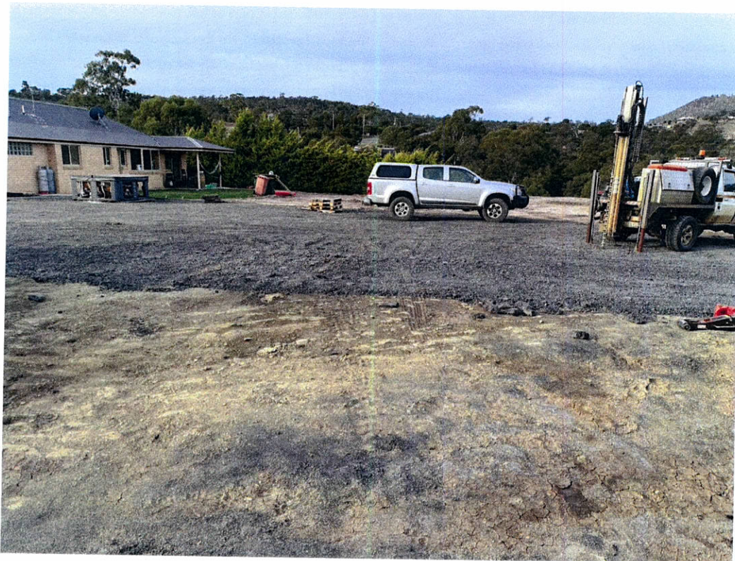
Plate 1 – Development site - looking across-slope to the southeast – Test Hole #1.
