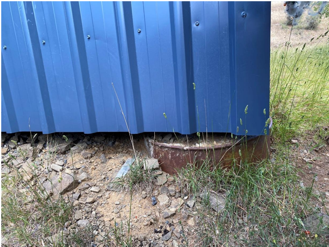
Figure 3: The footing at the NW corner of the shed/proposed dwelling. TH3 was completed to the side of this and refused at approximately 1.3 m depth on boulder fill/bedrock.
