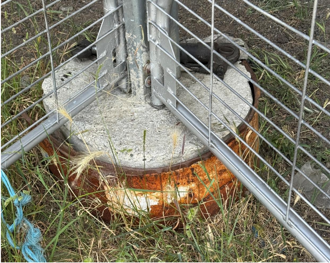
Figure 4: The footing at the centre southern side of the shed/proposed dwelling. DCP2 was conducted to the side of this and refused at approx. 0.1 – 0.2 m on multiple attempts.
