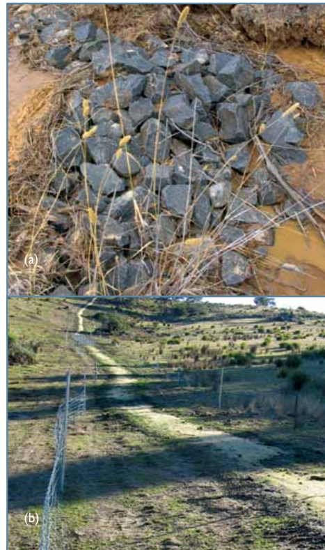
Figure 36. Examples of tunnel erosion control (a) Poor technique. Rock rap is usually an inappropriate erosion control technique for dispersive soils. Normally rock barriers work well to trap sediment and reduce erosion. However in dispersive soils, hard surfaces such as rock are quickly bypassed i.e. upper corner of the rock structure (b) Excellent technique. Note the entire repaired area is fenced, and the whole length of the repaired tunnel is covered with topsoil and jute cloth. Sand barriers have been constructed every 20 meters down the slope.
