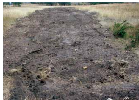
Figure 37. Good technique. Topsoil mounding, reclaimed tunnel erosion, Brighton. Note the width of earthworks required to fix a 50cm wide tunnel, and the raised profile to shed surface water. Jute cloth would prevent surface erosion until vegetation has established.
