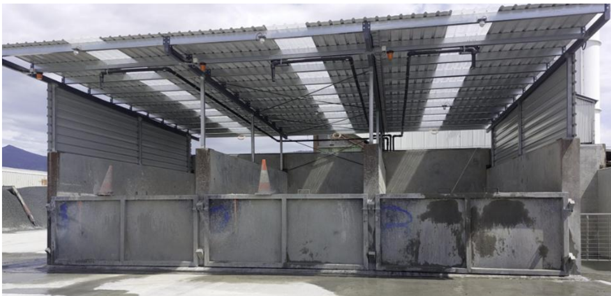
Figure 27. Example of covered wash out bays from Hazell Bros Lampton Avenue Batch Plant
