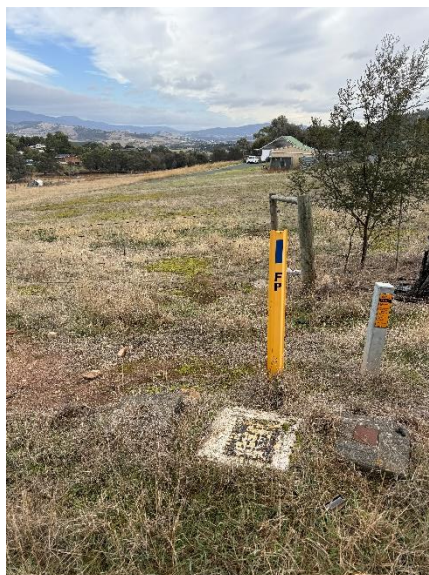
Figure 6 – Existing hydrant
