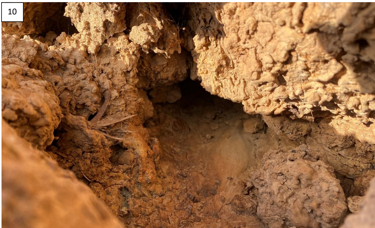
Photos 8-10: evidence of active tunnel erosion and clay dispersion in the nearby roadside cutting. This tunnel runs across the top of the flat sandy mudstone bedrock. Dribble patterns on all exposed clay faces. Fine sandy sediment fan deposits in an open table drain. See Figure 1 for photo locations.
