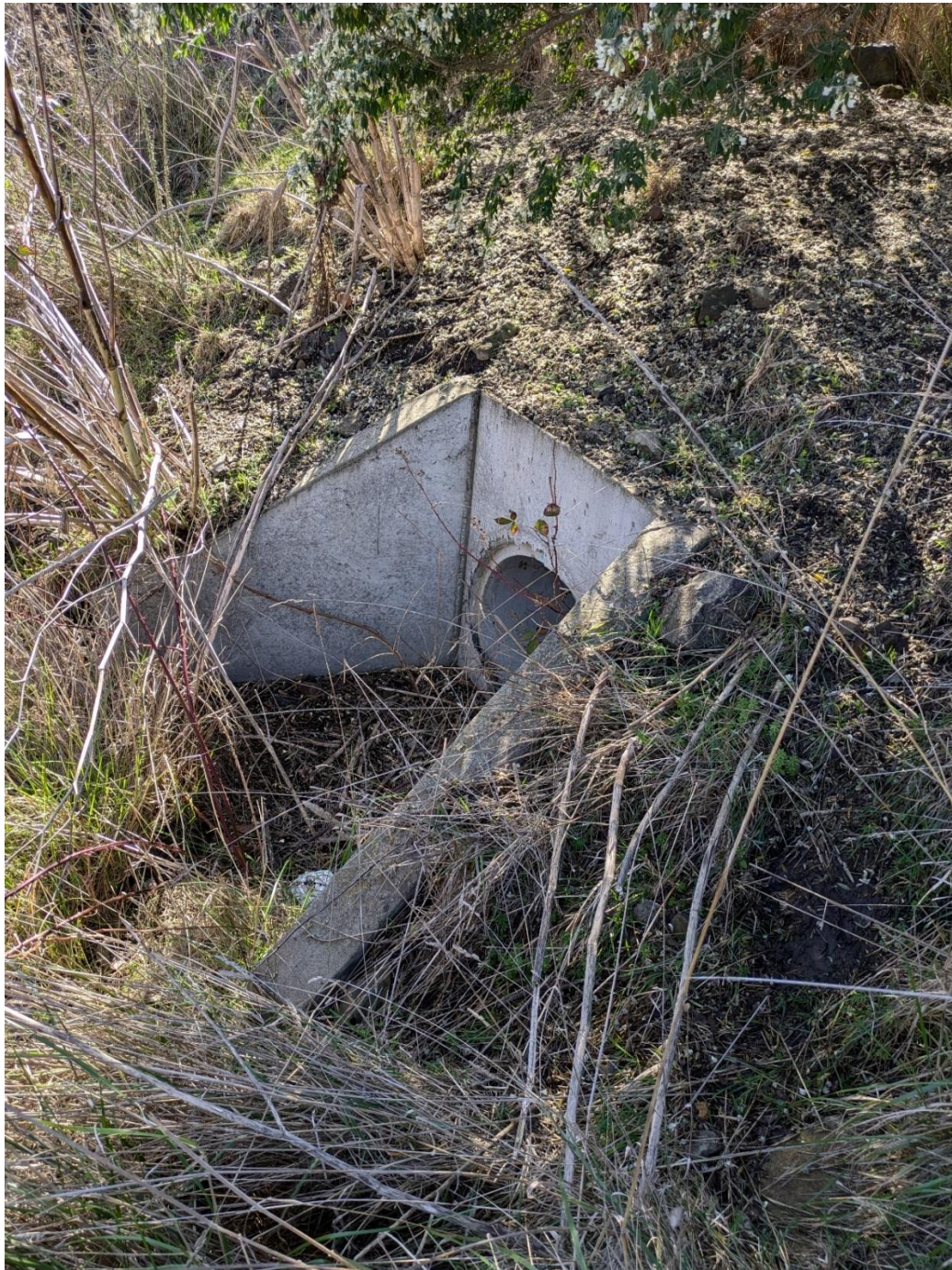
Photo of Department of State Growth Culvert Inlet Headwall and 750mm Pipe
