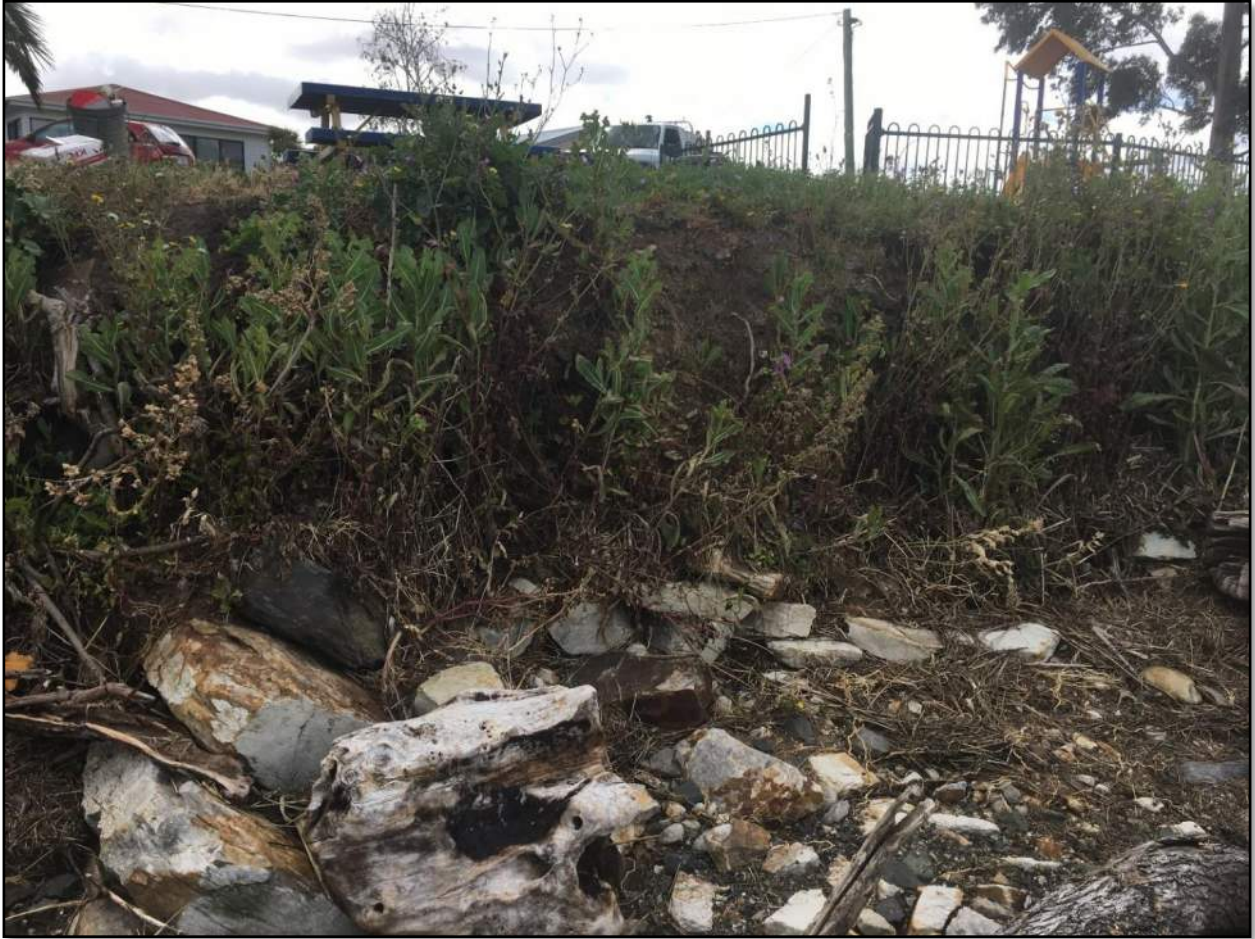
Plate 5 Fill Placed In Embankment Alongside Nielsen Parade
