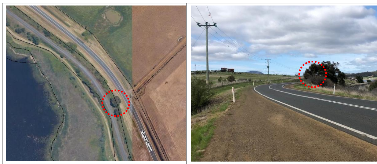
Figure 10 Access 3 Sight Distance - Vegetation Maintenance
