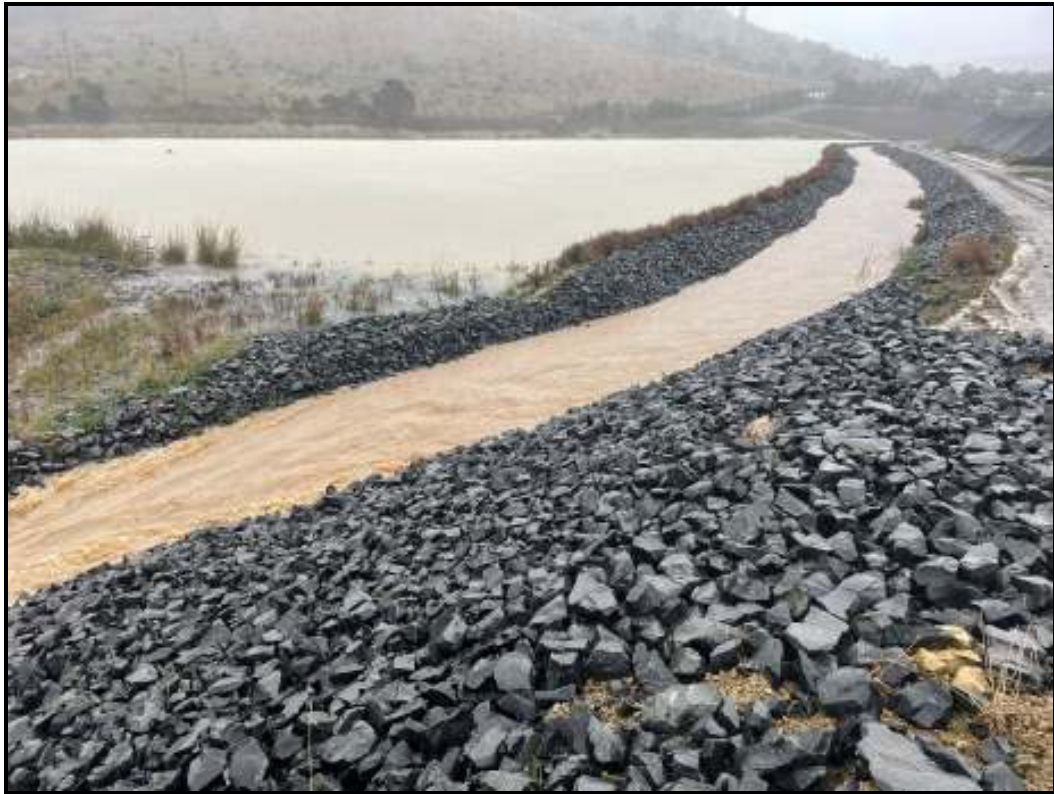
Water by-passing the dam during a very heavy rain-fall event
