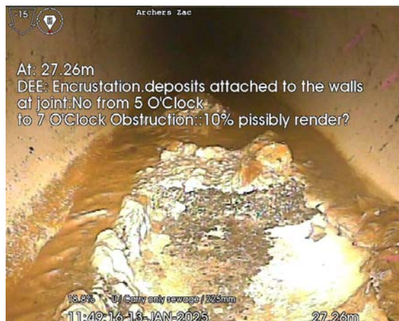
A360443_27-26m_114916.jpg, 00:03:53, 27.26 Encrustation-deposits attached to the walls from 5 o'clock to 7 o'clock, Obstruction: 10% / possibly render?
