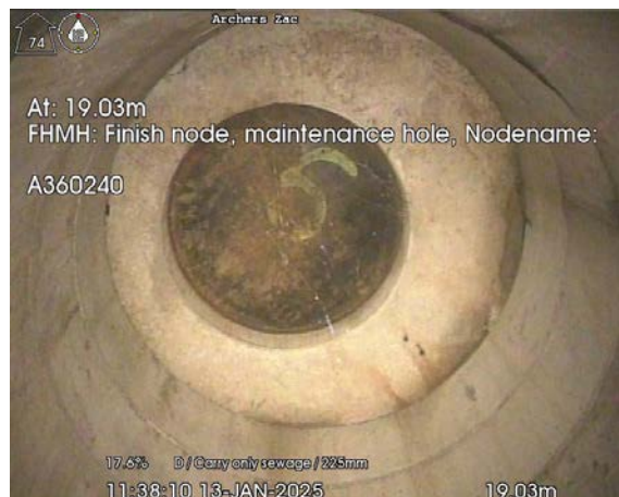
A360445_19-03m_113810.jpg, 00:03:06, 19.03 Finish node, maintenance hole, Nodename:, A360240
