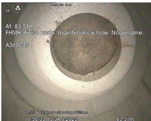
A360443_83-51m_115633.jpg, 00:10:55, 83.51 Finish node, maintenance hole, Nodename:, A360249
