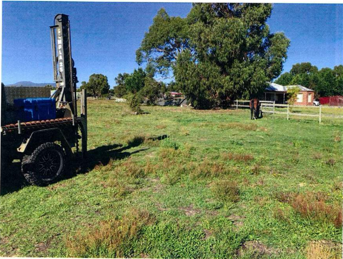
Plate 4 – Lot 2 – Test Hole #1.
