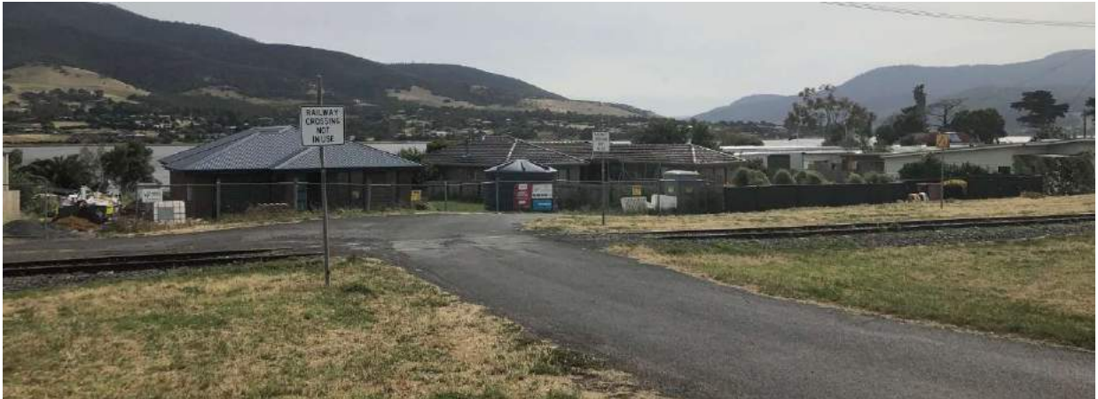
Figure 6 Wallace Street Derwent Valley Line Crossing
