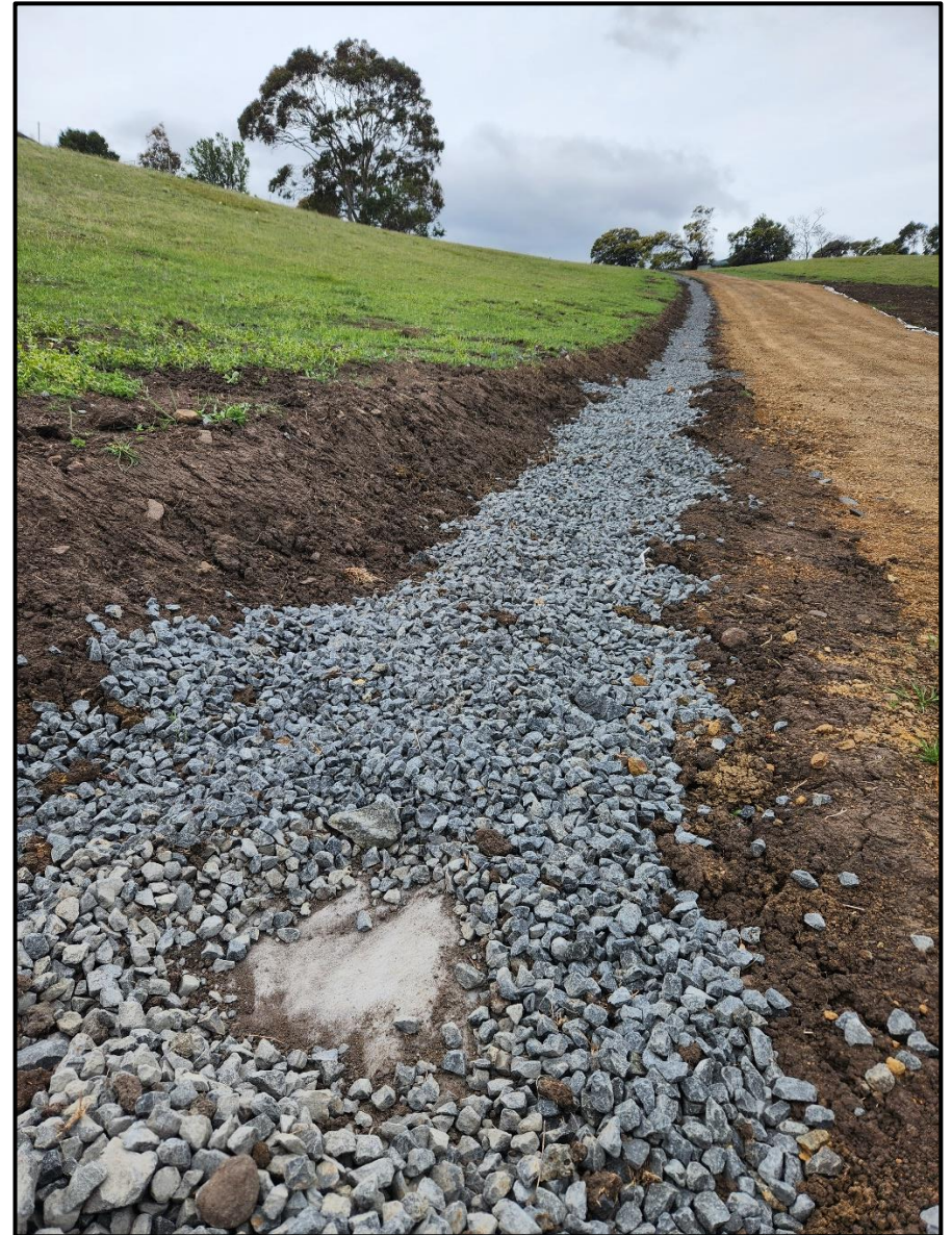
Photo 2 450x300, 100mm slotted pipe trench along driveway
