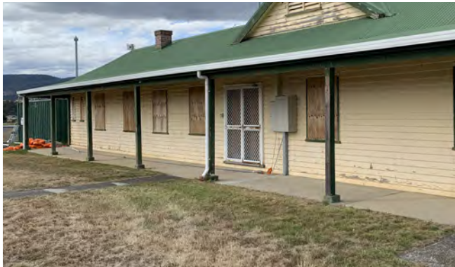
fig 9 Replacement of gutters and downpipes with more traditional profiles and materials is recommended. The external envelope is largely retained and refurbished. Subfloor ventilation should be provided.
