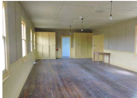
fig 5. Significant panelled wall, dado and ceiling linings, flooring and joinery are retained
