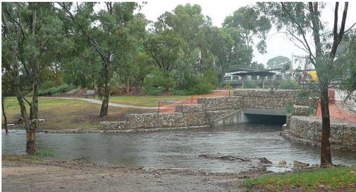
FIGURE 28: UNDERGROUND CULVERT IN BROWNHILL CREEK, SOUTH AUSTRALIA
