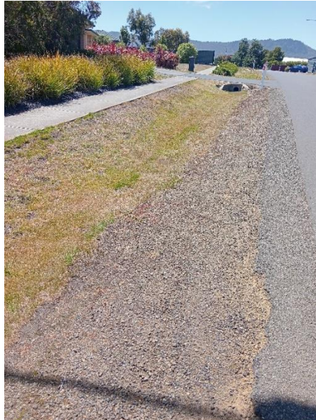
Figure 4 Storm water drains along Riviera Drive.
