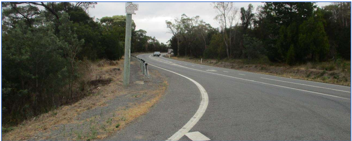
Photograph 5.2D – Available sight distance to the right at the southern junction
