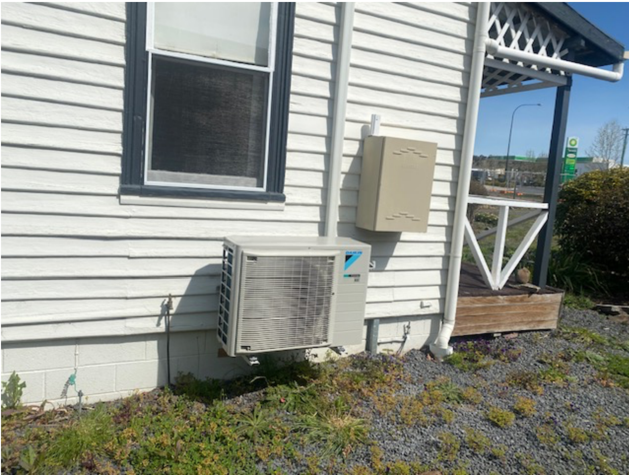
Photo 2 Relocated cottage now on Besser block foundations
