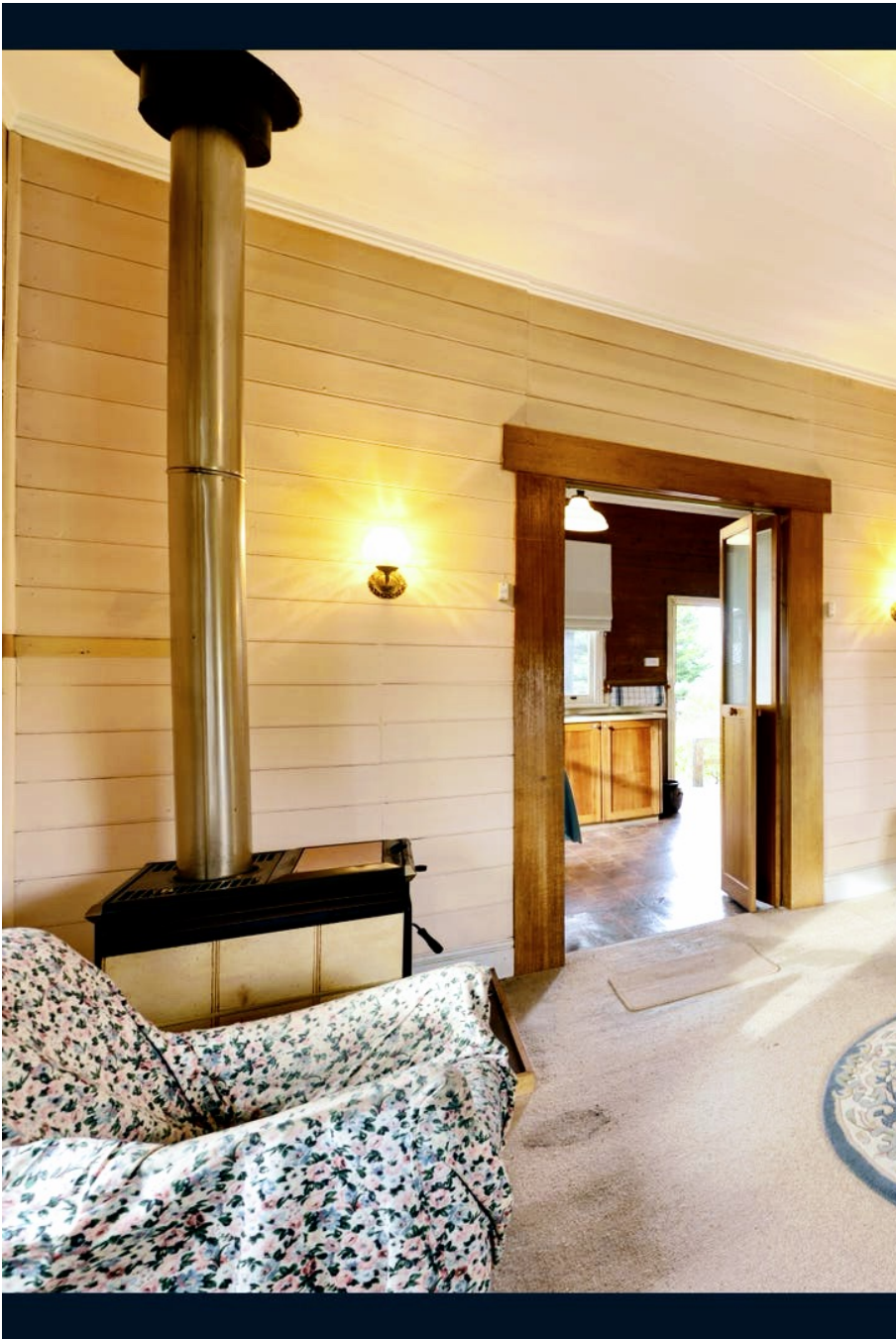
Photo 3 Internal view showing new doorway in original fireplace location
