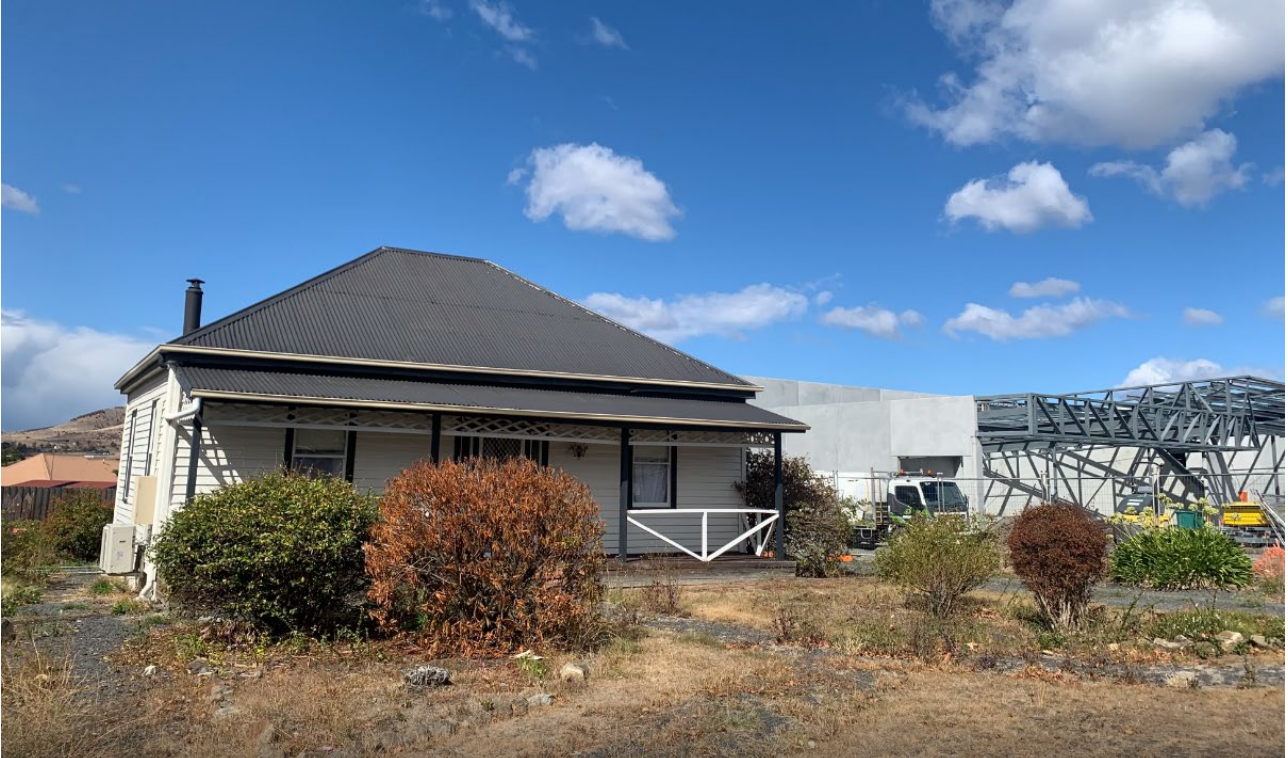
Figure 3 Photograph of the subject site, as viewed from Brighton Road. The site is located in the heart of the Brighton town centre, adjacent to the IGA development that is currently under construction, as well as the post office and pharmacy.
