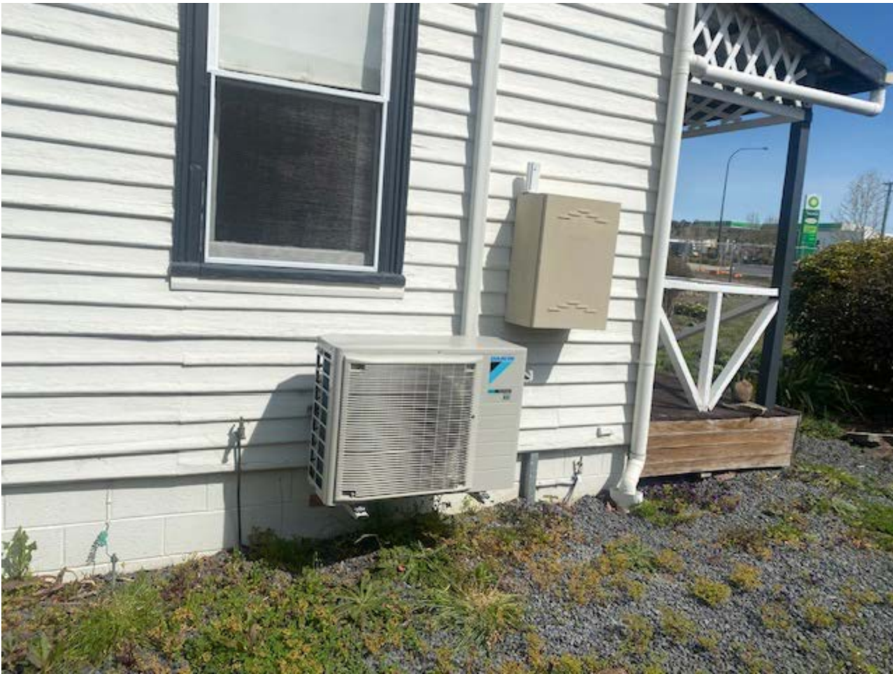
Photo 2 Relocated cottage now on Besser block foundations
