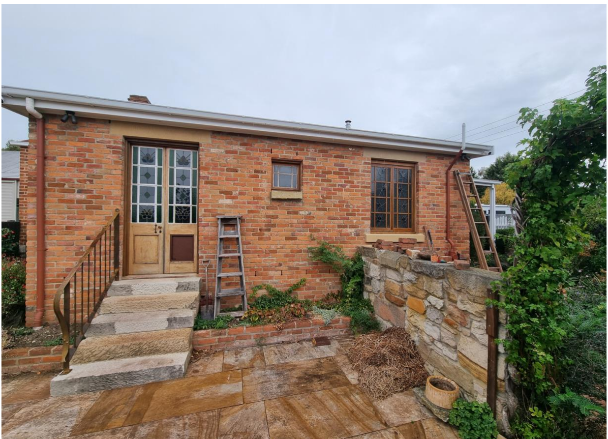
Figure 2 – The current rear of the cottage. Although this is not part of the original wall to the cottage, the pergola will be self-supporting and not actually fixed to the dwelling.
