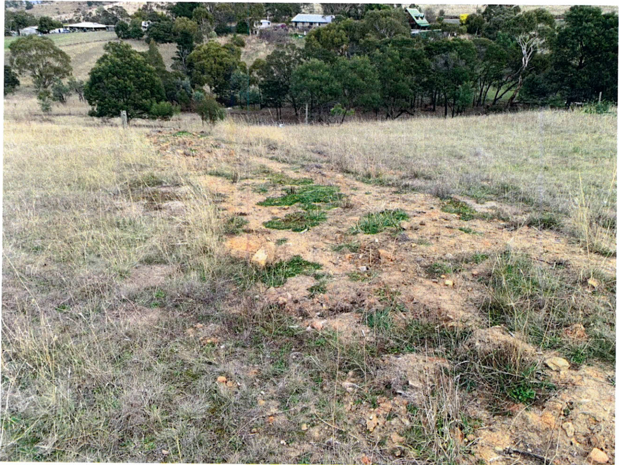
Plate 4 – House site – looking downslope to the southwest, area of tunnel / open erosion that has been infilled
