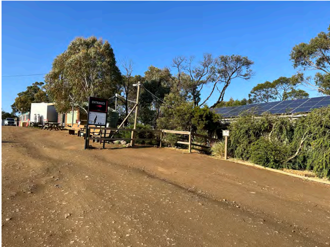
Fig 26. The existing site of the proposed new expanded veterinary hospital.
