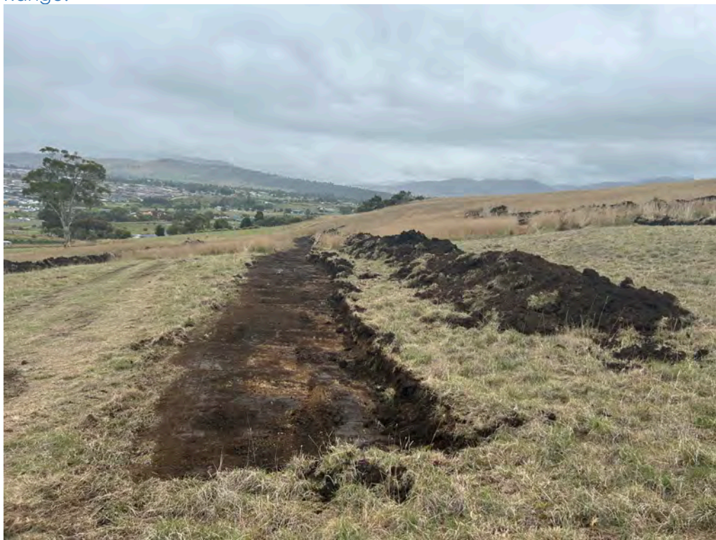
Fig 35. New landscaping swales to aid in hydrology and a new tree planting program to encourage wildlife and redevelop wildlife corridors between the Jordon River and the Meehan Range.
