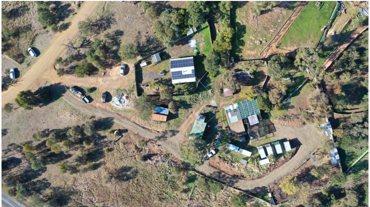
Fig 13. Aerial of the back of house shed and facilities close to Briggs Road.
