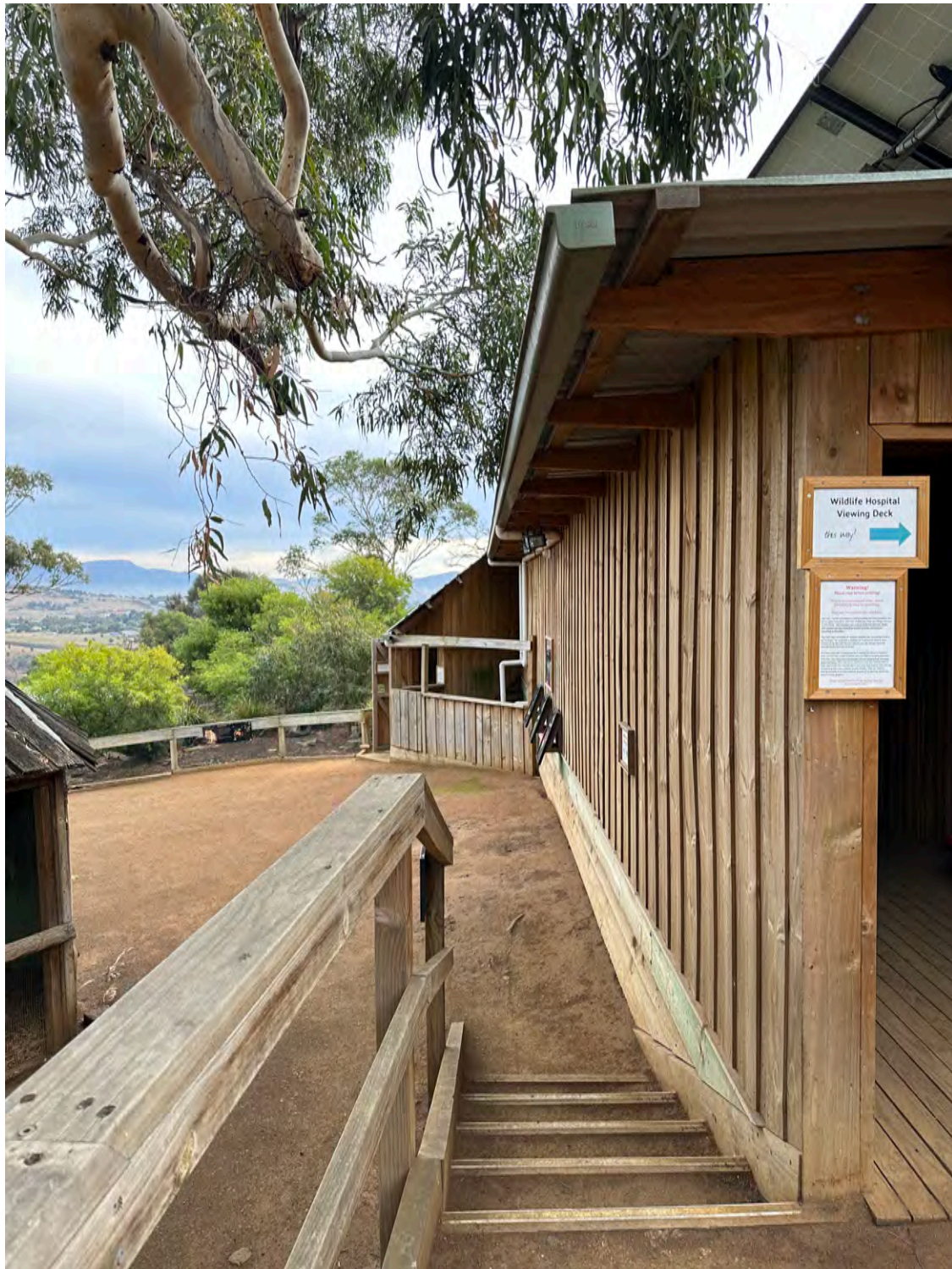
Fig 22. The new ramps will allow wheelchair access and walking frames and prams. The ramp will aid in moving across the undulating terrain.
