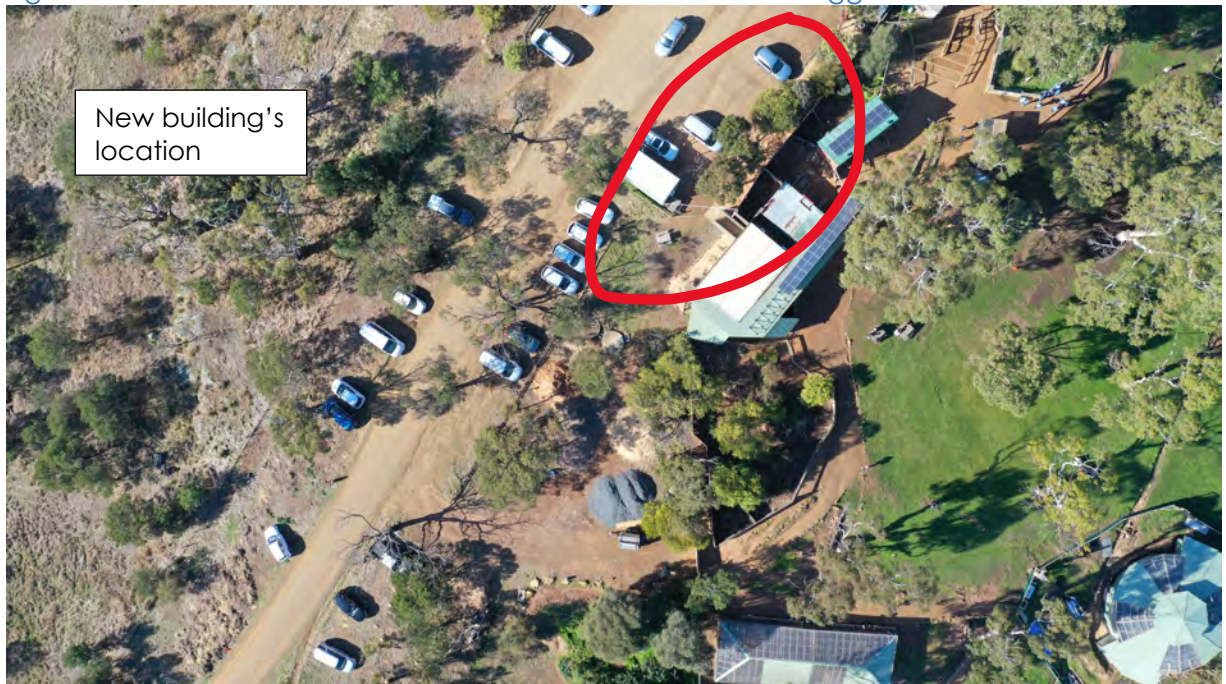
Fig 14. Aerial image of the car parking and the location of the proposed expanded veterinary hospital.
