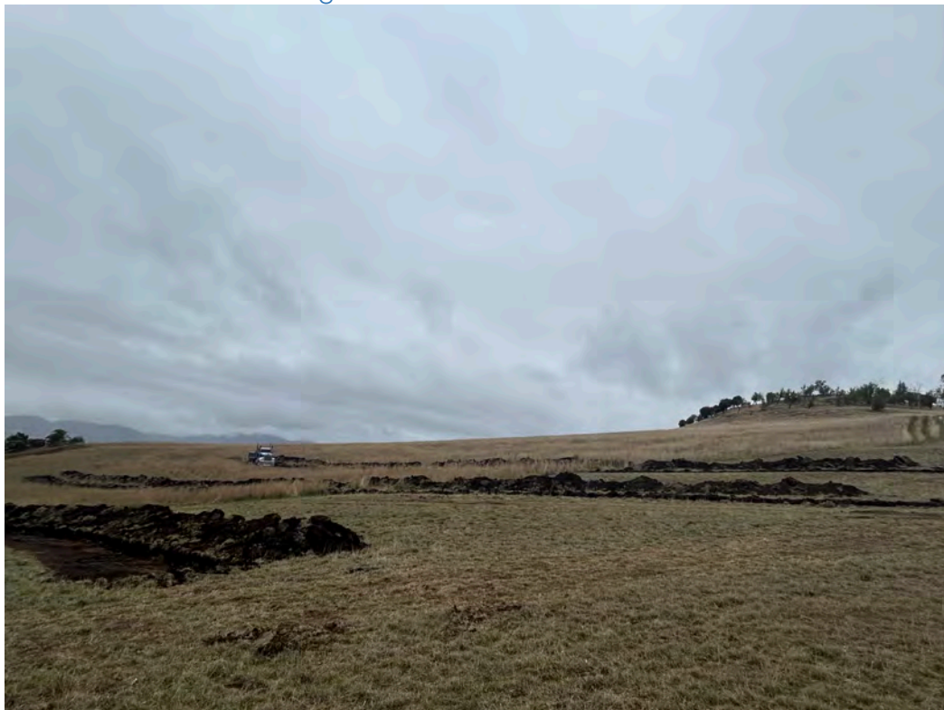
Fig 33. Working with McConnell Dowell, the builders of the new Bridge Water Bridge, Bonorong is using local stone to create new landscaping swales to aid in hydrology and a new tree planting program to encourage wildlife and redevelop wildlife corridors between the Jordan River and the Meehan Range.
