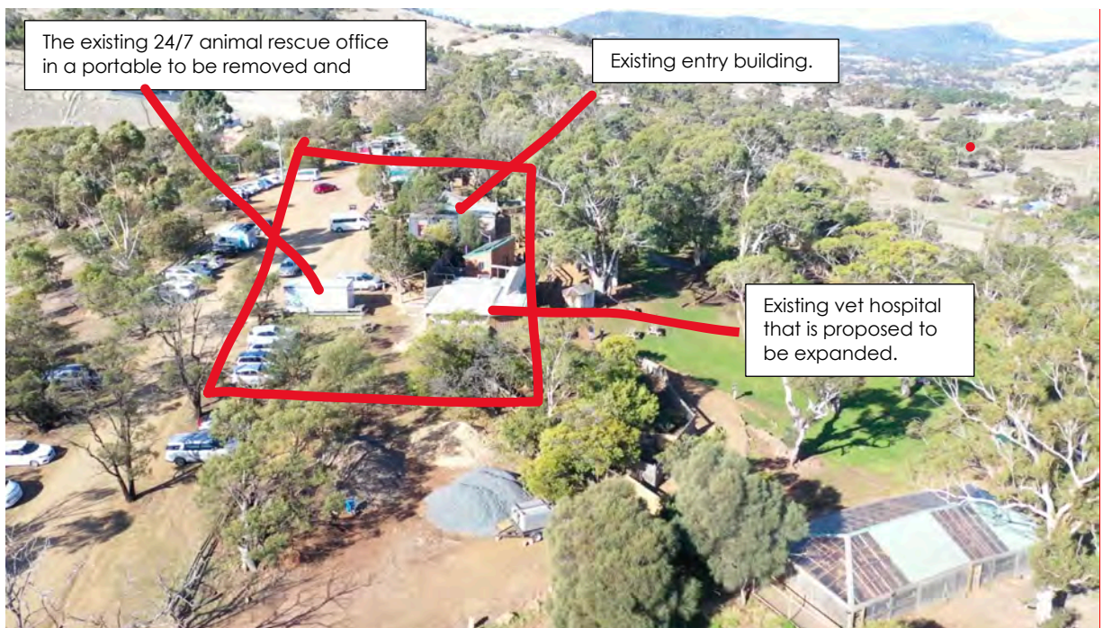
Fig 6. Looking at the existing vet hospital, the 24-hour rescue portable, and the location of the proposed expanded vet hospital.
