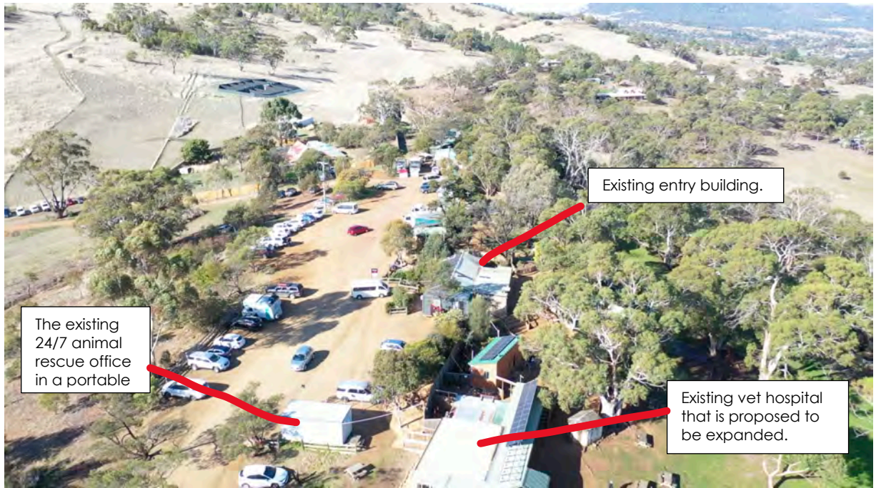
Fig 7. Looking north across the site.
