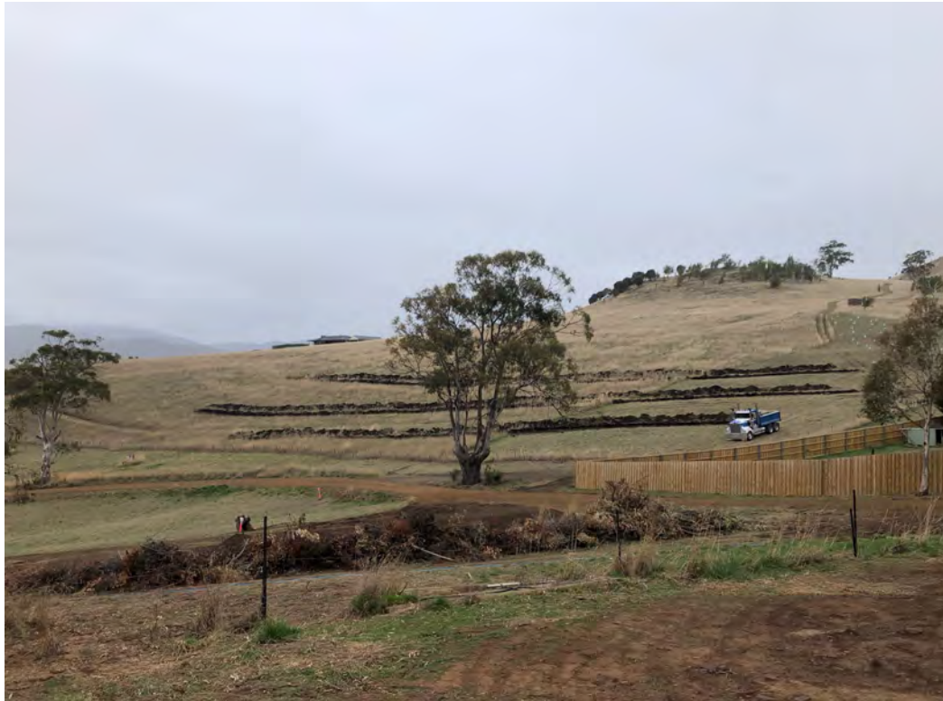
Fig 32. Working with McConnell Dowell, the builders of the new Bridge Water Bridge, Bonorong is using local stone to create new landscaping swales to aid in hydrology and a new tree planting program to encourage wildlife and redevelop wildlife corridors between the Jordan River and the Meehan Range.
