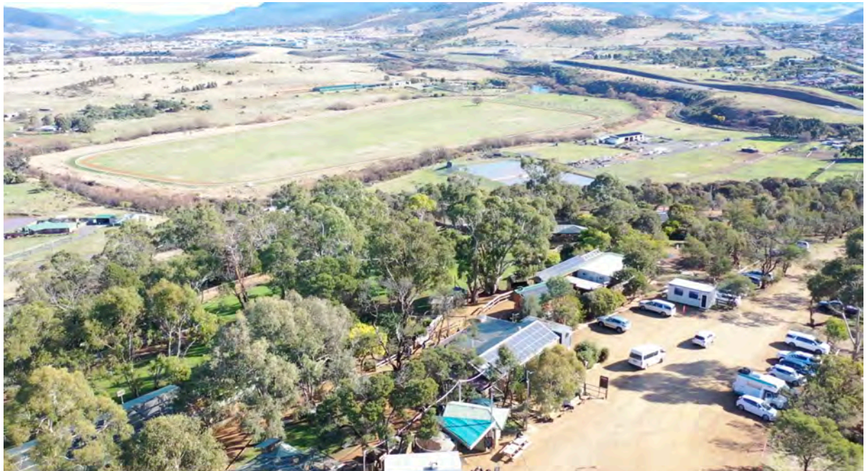
Fig 4. Looking northwest across the existing Bonorong car park and entry to the sanctuary.
