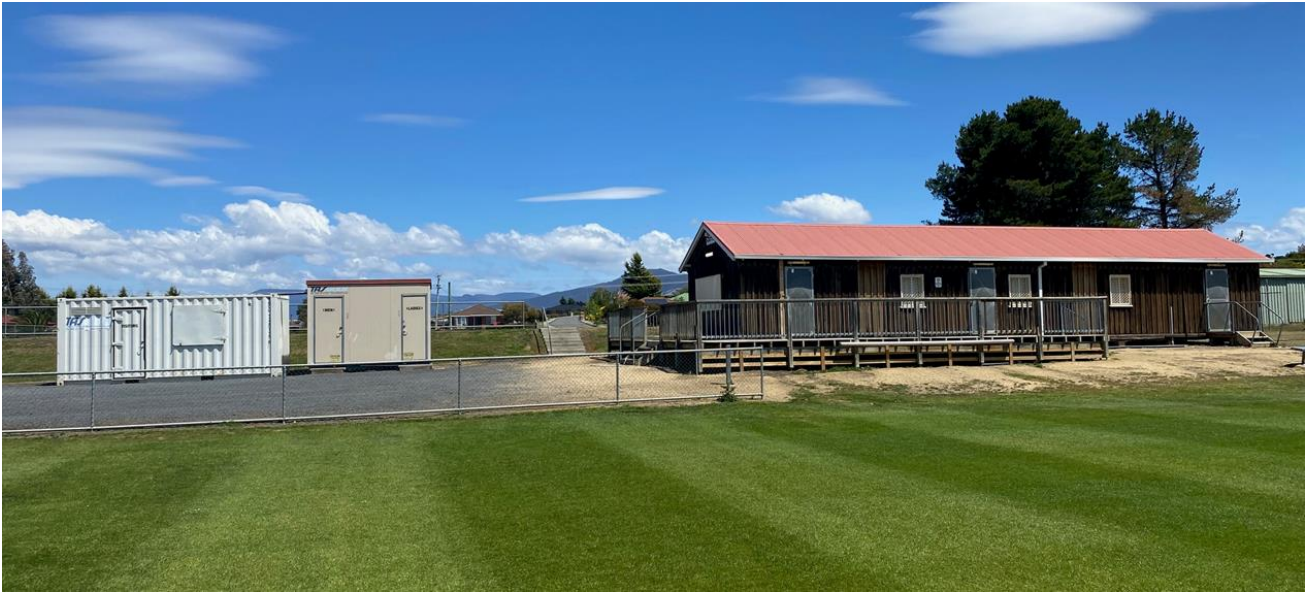
Figure 2 – Existing buildings to be removed from the site (Source: Brighton Council)
