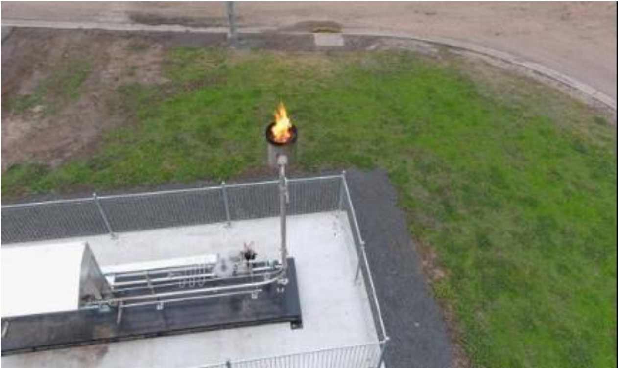
Figure 4: an image of the biogas flare to be installed at Green Point STP.
