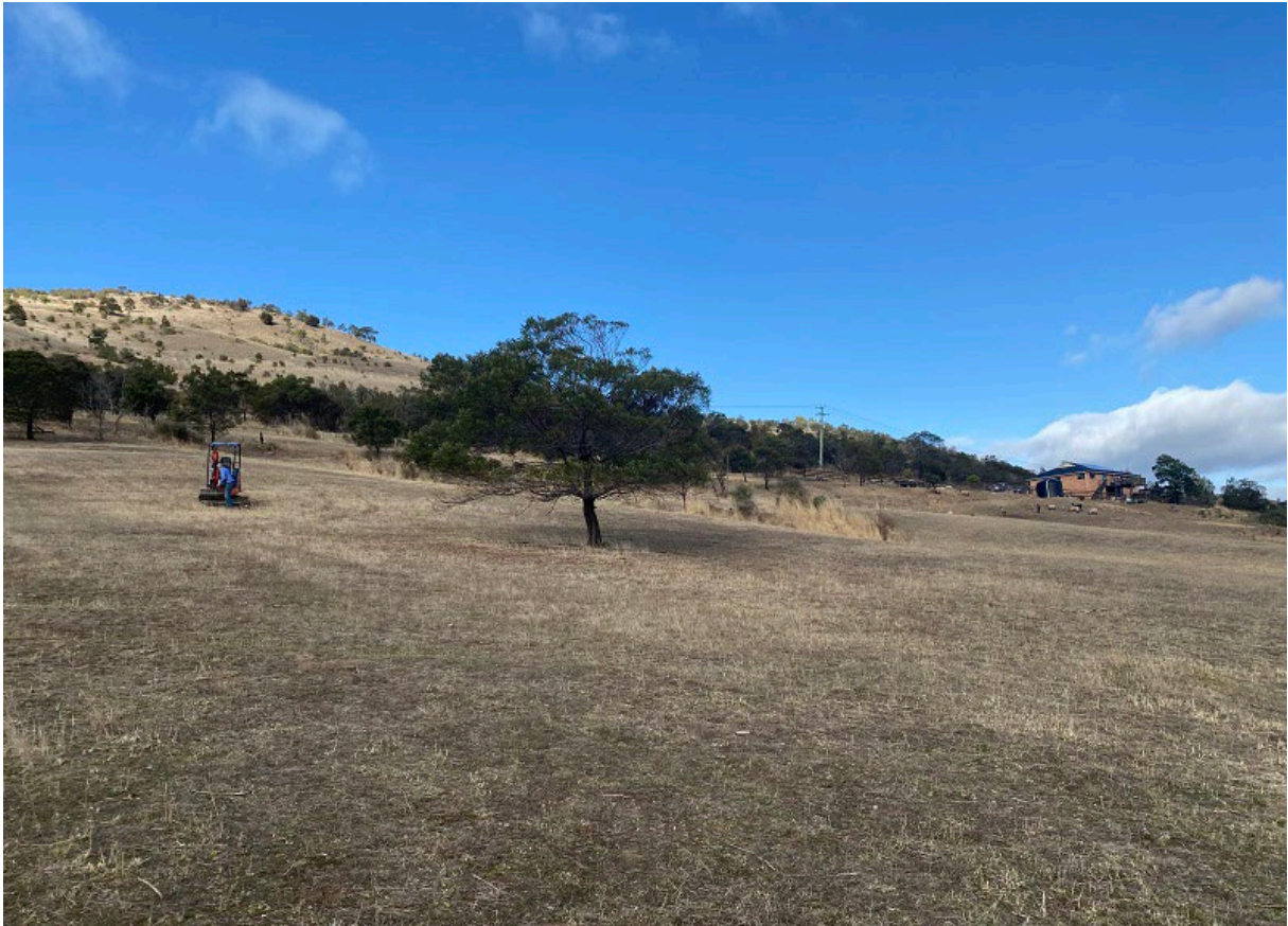
Plates 5 (above). View diagonally upslope on proposed Lot 2 to the southwest, from near the lower northeastern property corner. The excavator is digging test pit B.
