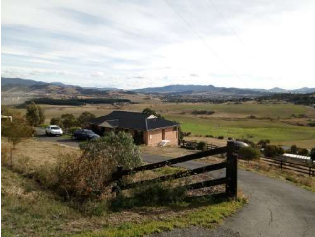
Image 3: Looking northwest towards Lot 1.
