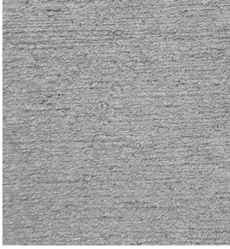
BROOM FINISHED CONCRETE DRIVE/ CARPARKS
