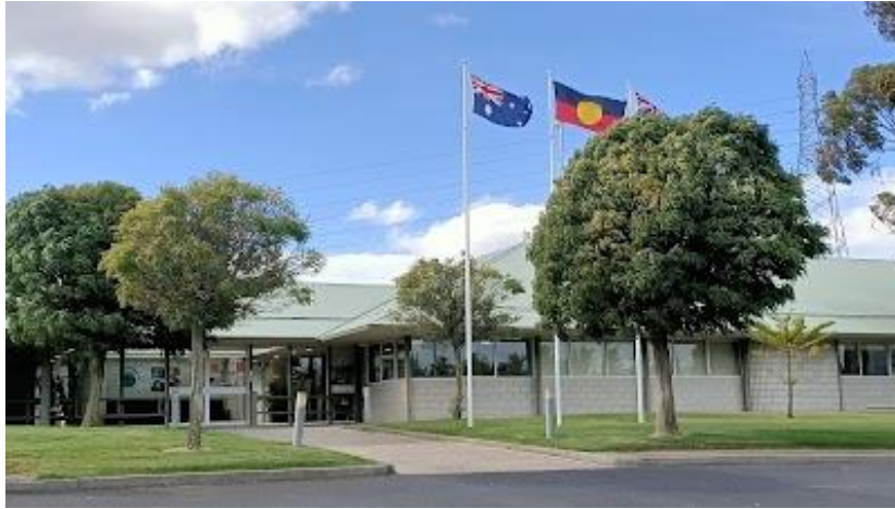
Figure 16 Brighton Council Chambers
