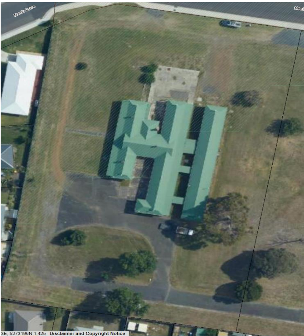
Figure 2: Aerial image of site (source: www.thelist.tas.gov.au )
