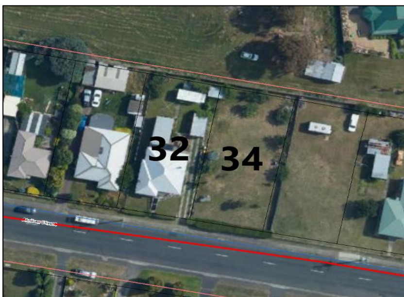
Figure 1. An aerial image of the site and its immediate surrounds
