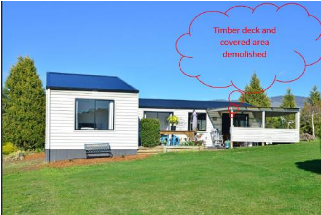
Figure 4 View of unapproved covered deck (Source RealEstate.com Aug 2020)
