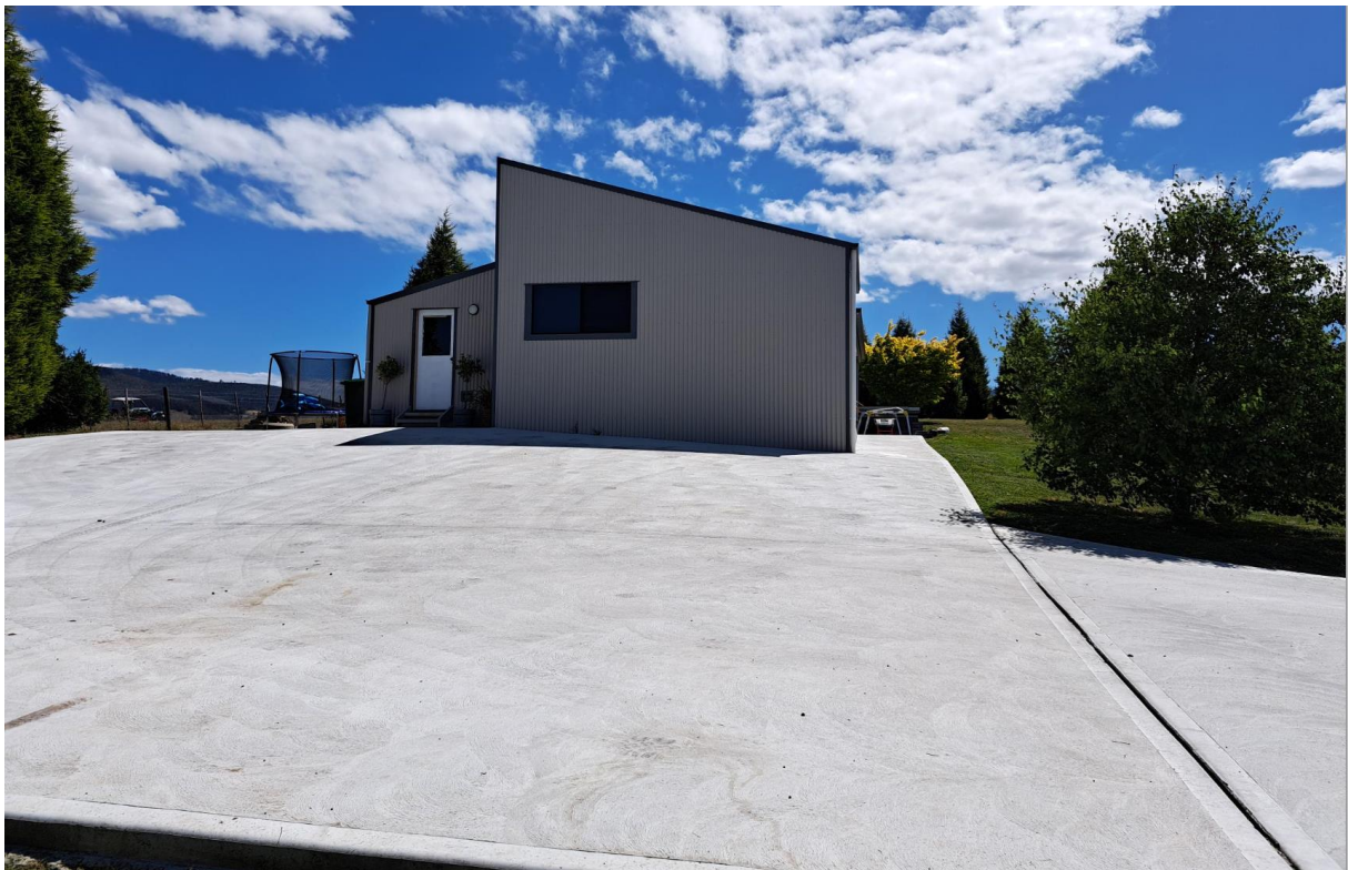
Figure 9 Image of completed works - East elevation (Source: IBoss - December 2022)
