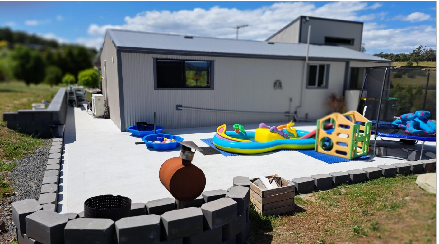
Figure 8 Image of completed works - South elevation (Source: IBoss - December 2022)
