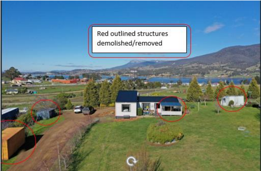
Figure 2 Aerial view of existing development prior to settlement (Source RealEstate.com August 2020)
