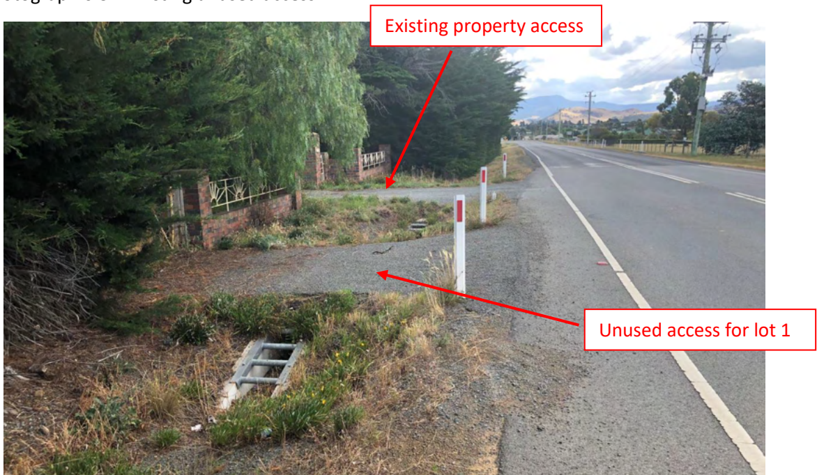
Photograph 6.3 – Existing unused access
