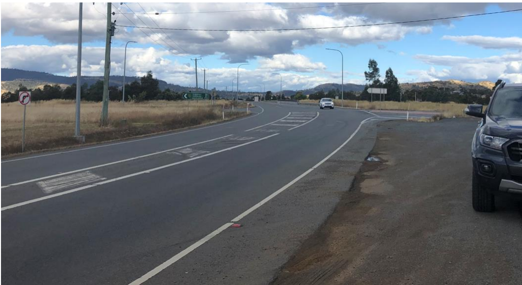
Photograph 6.4B – View looking east from the proposed lot 2
