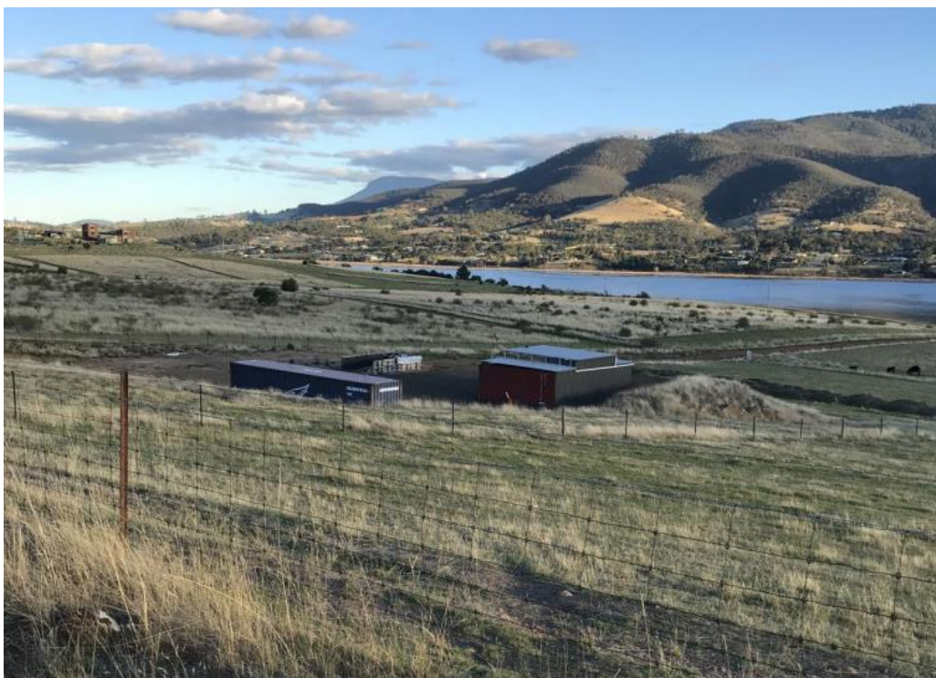
Photograph 1. Taken north of site showing recent earthworks and outbuildings
