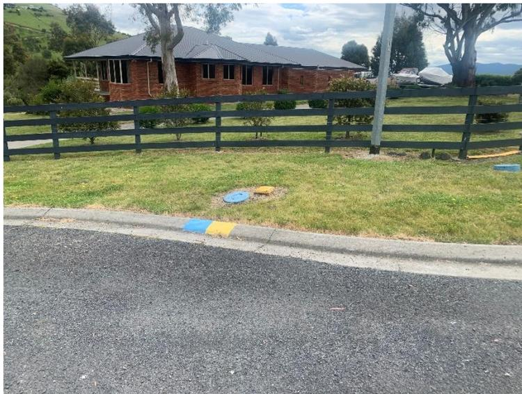
Figure 7 Existing fire hydrant (not shown on *The LIST Map*)
